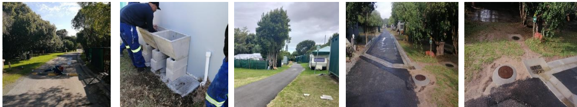
Maintenance work was done to upgrade facility
