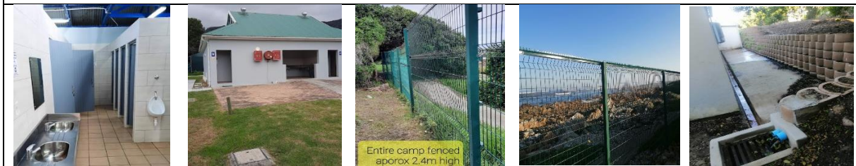
Speedbumps, wash basin and Taring road
